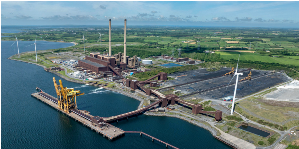
Figure 2: Moneypoint Power Station
