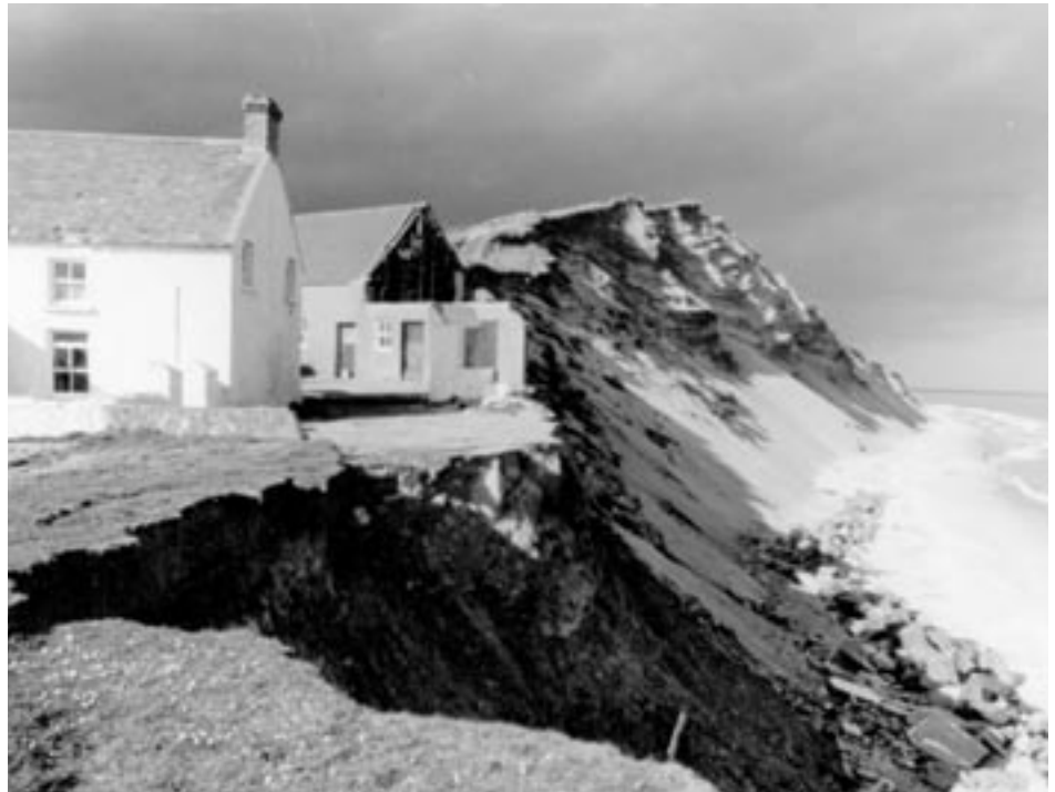
Coastal erosion is already a serious problem along the sandy Blackwater coast of Co Wexford. But by 2100, the rate of coastal erosion around Ireland could be three or even four times faster than today.
