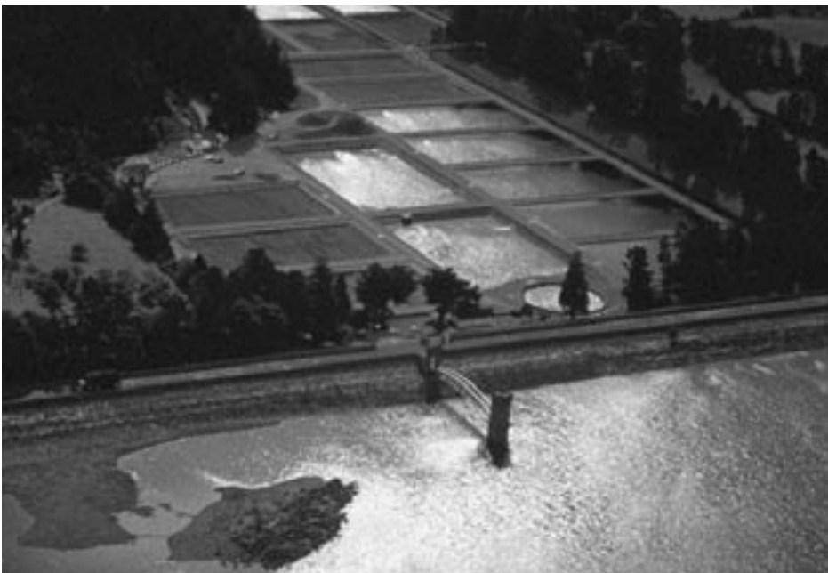
Drinking water treatment plant at Roundwood, Co Wicklow. Currently, 70% of Ireland's water supply comes from such surface water, but where will we get our water when climate change takes effect?
