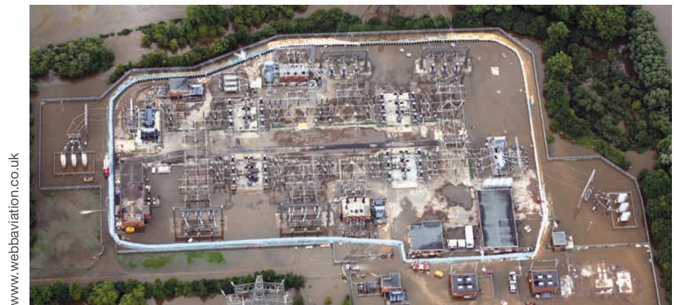
Walham electricity substation, Gloucestershire, July 2007: a temporary barrier (blue) kept peak flood waters at bay, but the crisis came within inches of a blackout that would have affected 500,000 homes, hospitals, critical infrastructure and industry.
